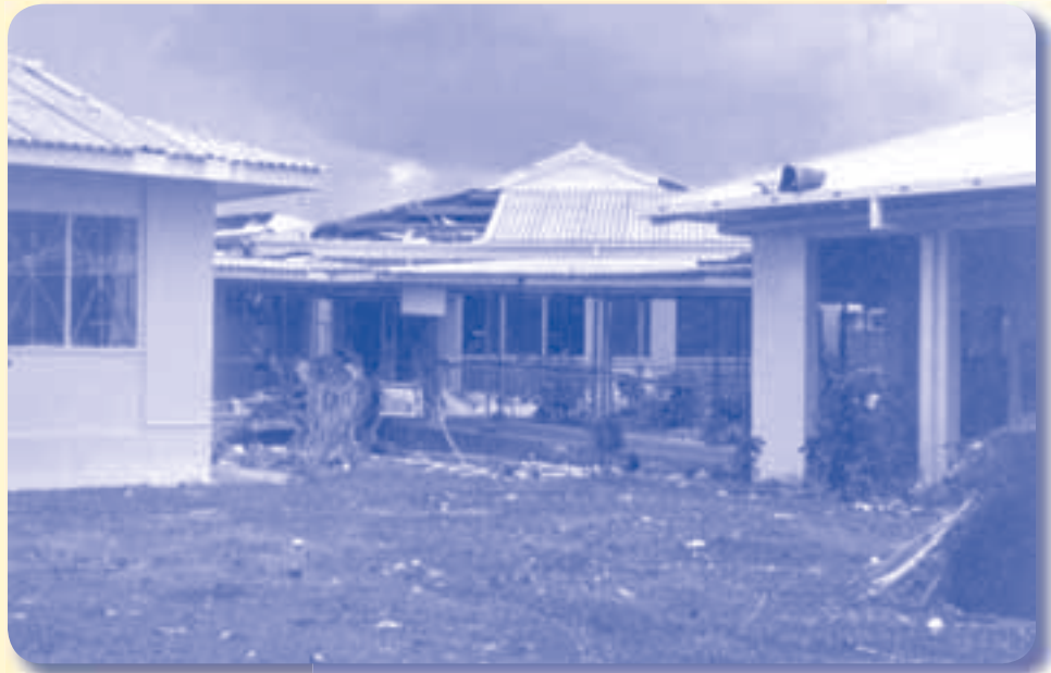
NTRS 1655, Mrs P. Hart collection, item no. 10, view of Darwin hospital buildings
